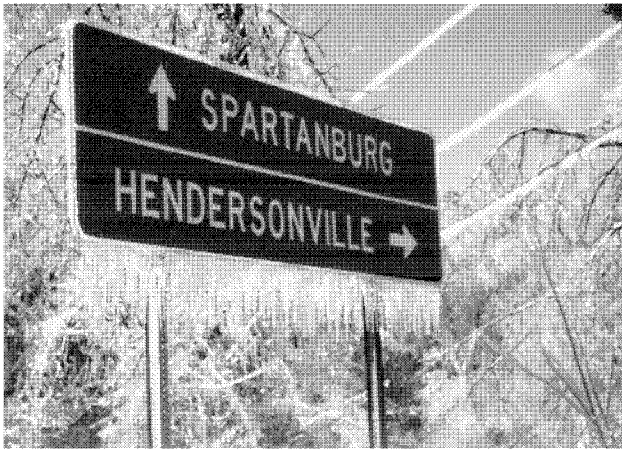
FIGURE C10-1 GLAZE ICE ACCRETION DUE TO FREEZING RAIN
